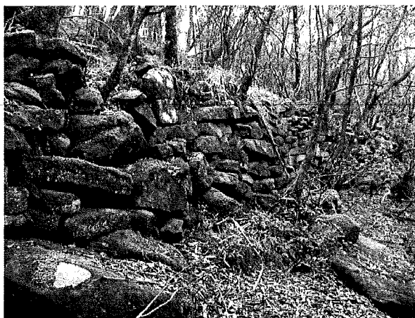
Figure 5. Mill race, retaining wall along west side (courtesy of KCHS)
