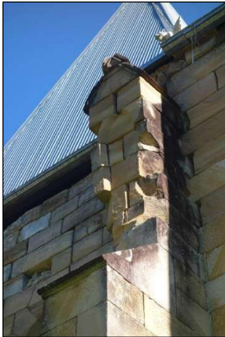
P05 – TYPICAL DAMAGE TO STONE BUTTRESSES
