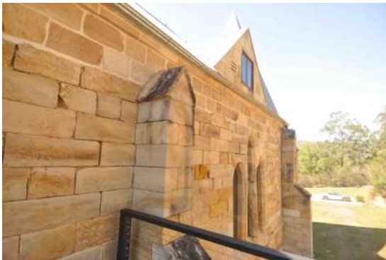
Figure 77: View of the mortar joint failure on the western elevation.
