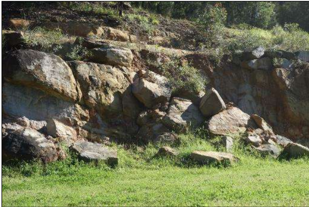
P13 – LANDSLIP IN BEDROCK/ BOULDER TERRACE WALL
