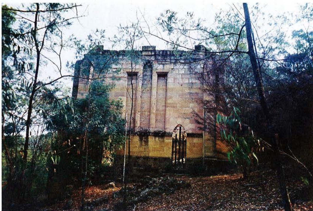
Figure 6: Photograph of the north façade showing window to the rear of the altar, arched doors on either side of the window and indications of a gable roof.
