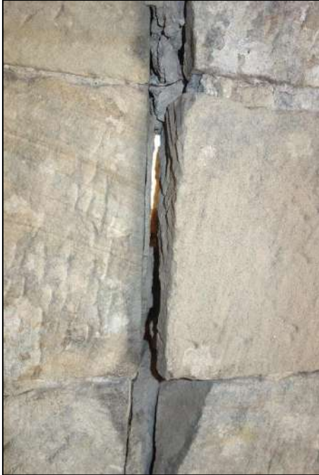
P09 – TYPICAL OPEN MORTAR JOINT
