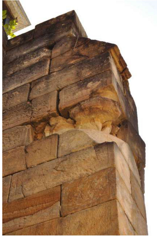
Figure 76: View of advanced localised exfoliation on the buttress to the western elevation.
