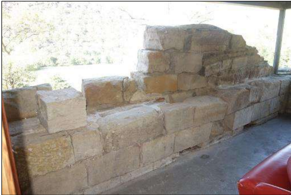
P11 – LOOSE STONES AT TOP OF WALLS
