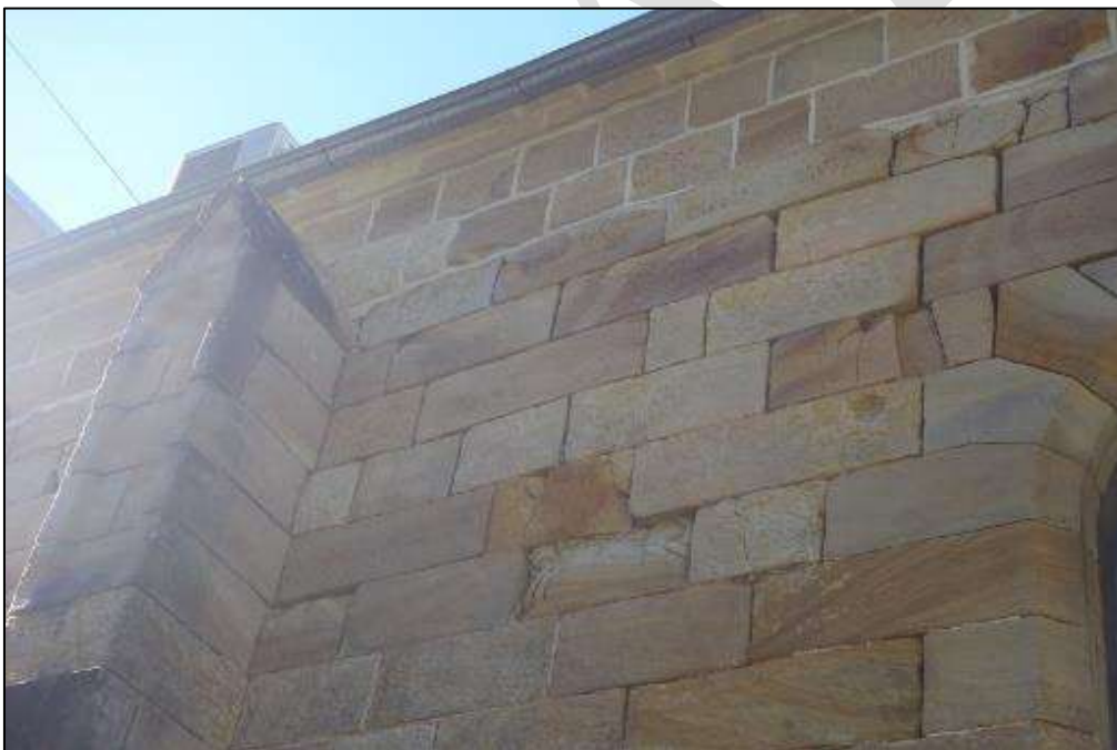
P04 – TYPICAL CRACKING AND EROSION OF STONEWORK
