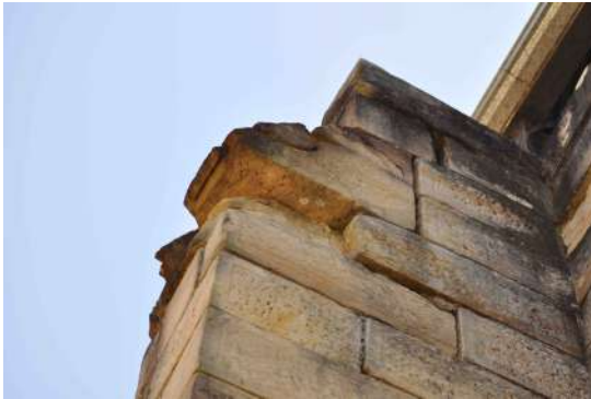
Figure 69: View of the disaggregation of stone blocks to the upper portion of the buttresses.
