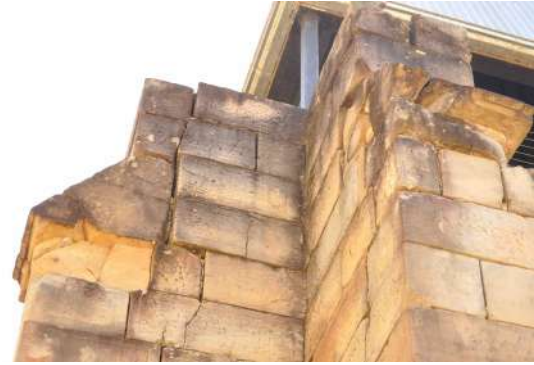
Figure 68: View of the failure of mortar joints and failure of stone blocks with vertical cracking.
