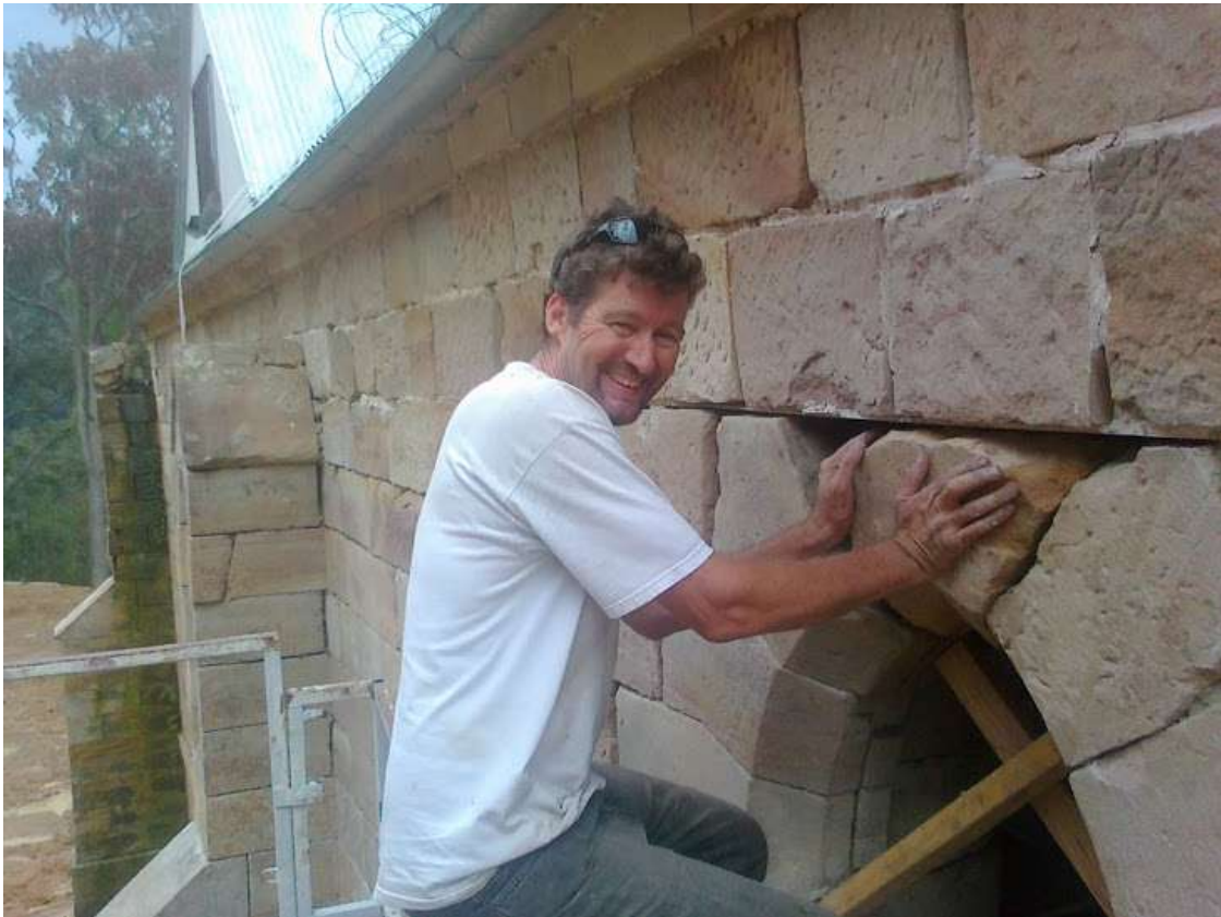
Figure 19: View of Steve Kavanagh completing the lancet window reconstruction to the western side elevation.
