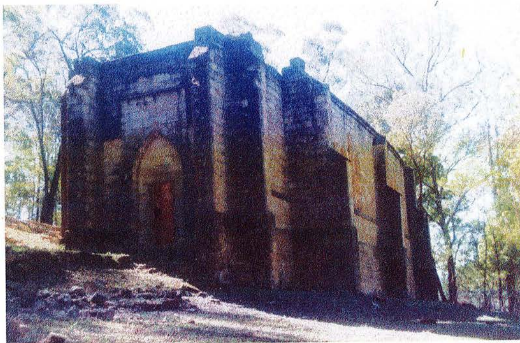
Figure 11: Photograph showing extent of rotation and bow in east façade (Photograph: John McInnes, February 2003).
