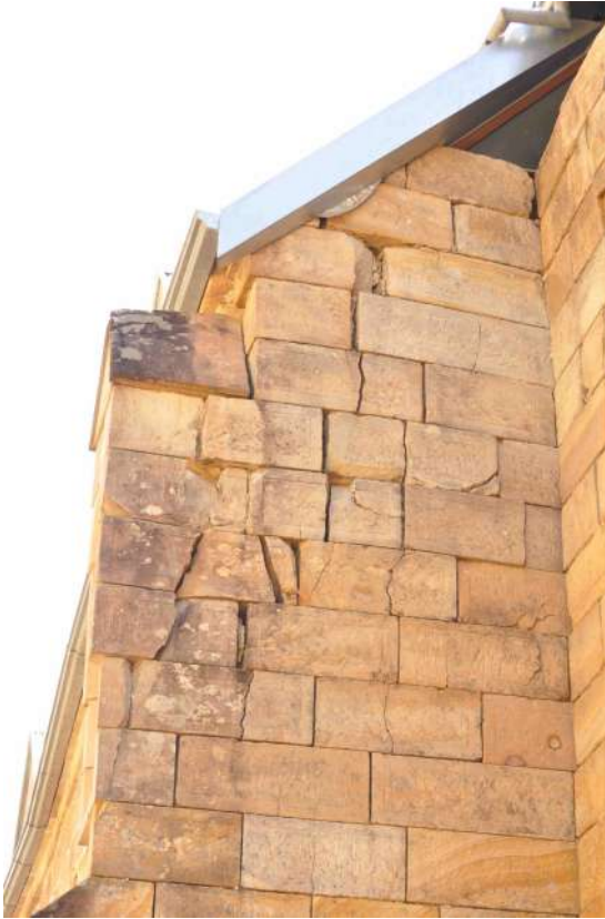
Figure 75: View of mortar joint failure and stone block failure to the buttress on the western elevation.
