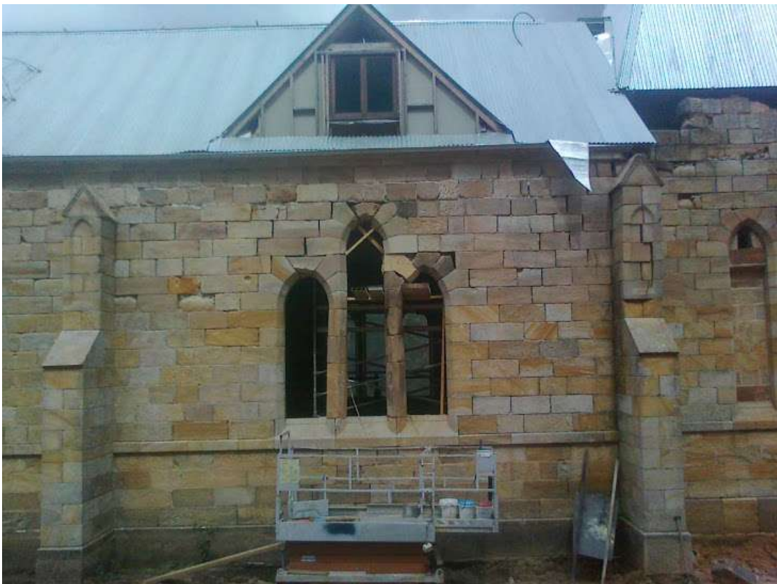
Figure 20: View of the completed lancet window reconstruction to the western side elevation.
