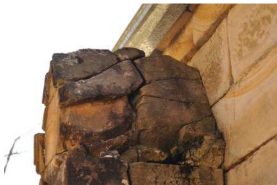
Figure 80: View of the disaggregation to the bolection on the western side buttress.
