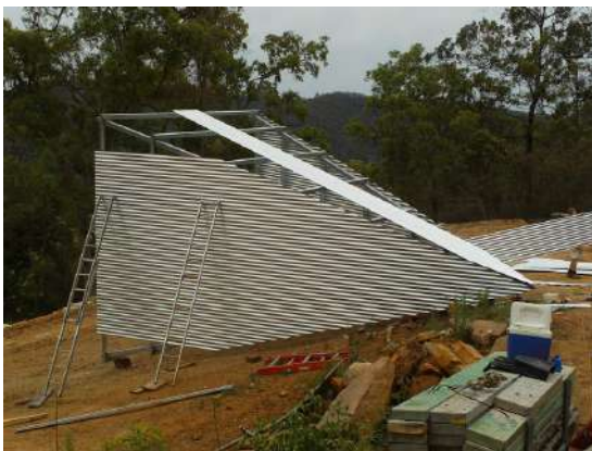
Figure 16: View of the new steel spire under construction.
