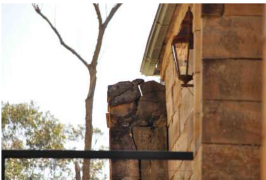
Figure 79: View of the disaggregation to the bolection on the western side buttress.
