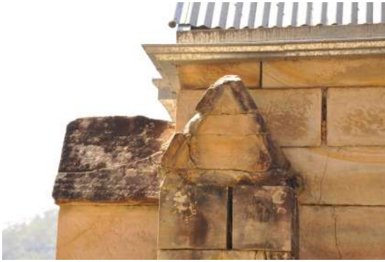
Figure 81: View of the disaggregation to the bolection on the western side buttress.
