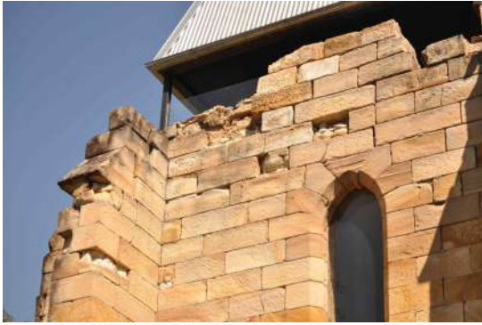
Figure 67: View of the upper walls of the tower structure showing displacement of stone blocks and disaggregation.
