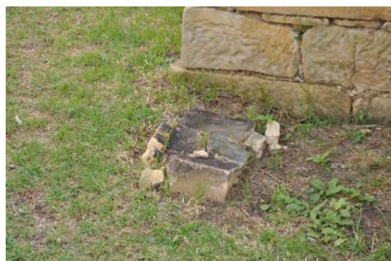
Figure 74: View of recent delaminated stone blocks on the western elevation.
