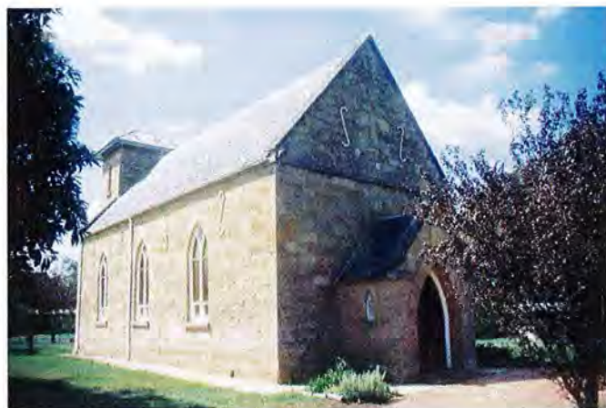
Figure 5. St. Bede's Catholic Church, Appin, NSW. The original crenellated top portion has been removed from the tower which has been re-roofed in galvanised steel.
