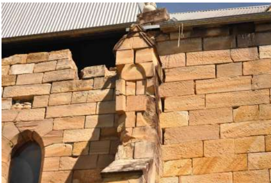
Figure 71: View of the buttress and upper portion of the eastern wall showing displacement of stone blocks.
