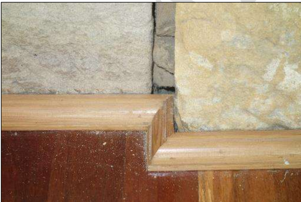
P10 – EVIDENCE OF ONGOING FRETTING STONE/ MORTAR (STONE DUST ON FLOOR)
