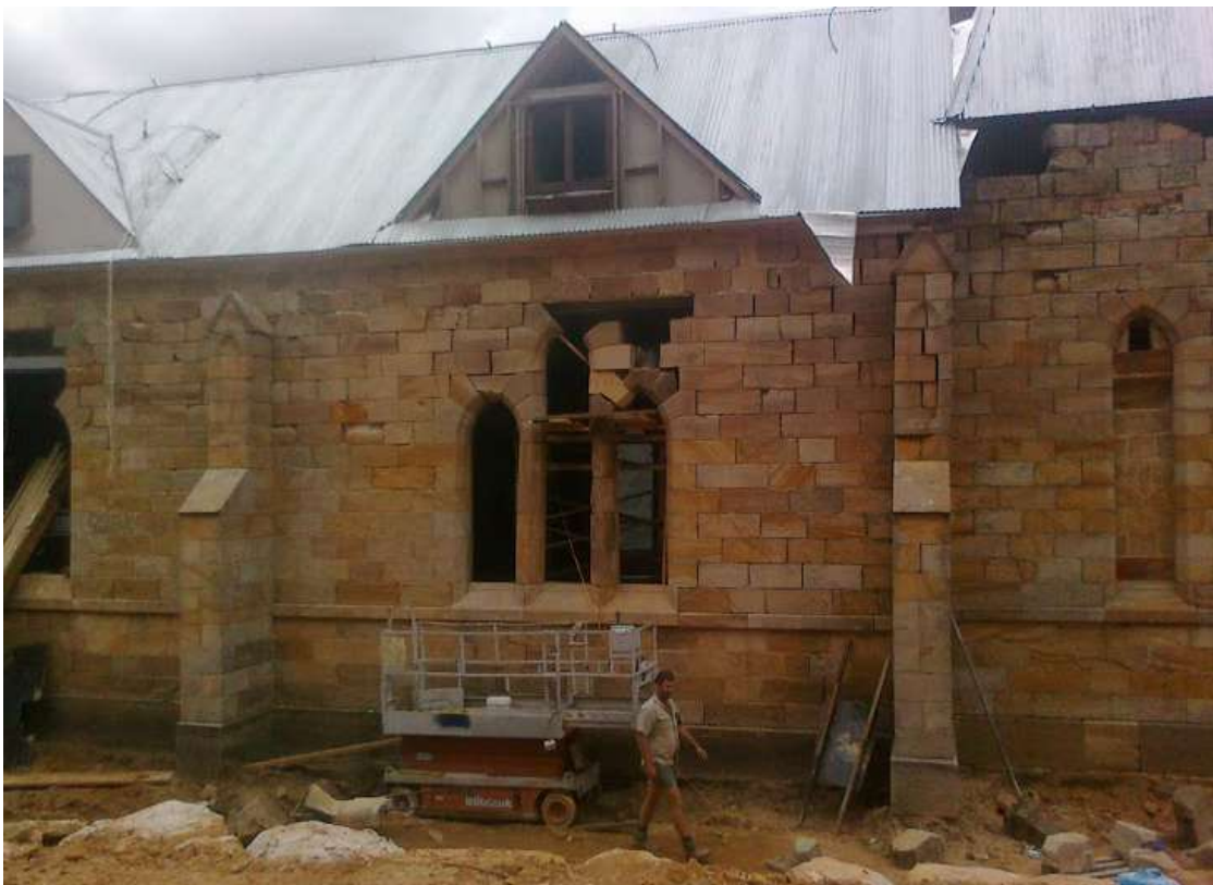
Figure 18: View of the western side elevation during reconstruction of the lancet windows.
