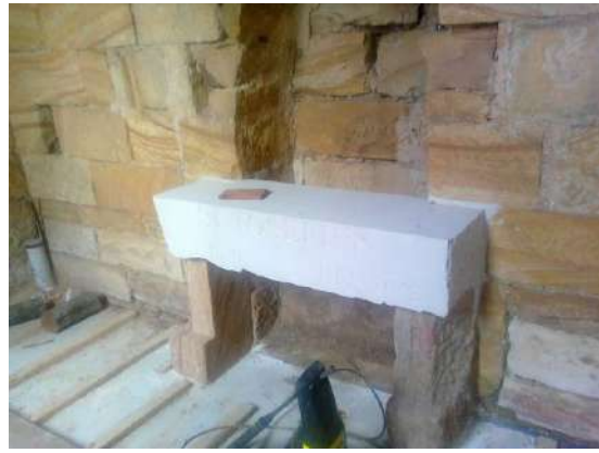
Figure 15: View of the replacement lintel to the fireplace in the lobby.
