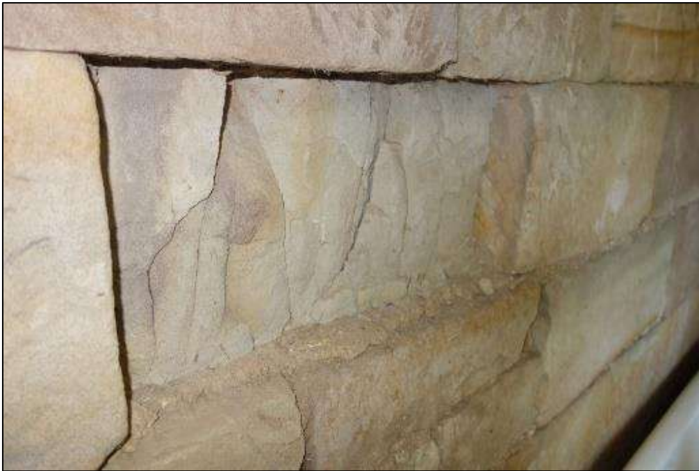
P07 – TYPICAL FRETTING OF STONES (INTERNAL FACE)
