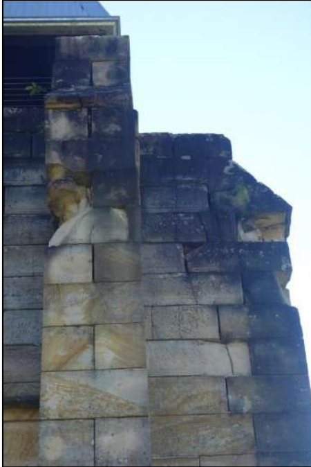
P03 – TYPICAL DETERIORATION OF BUTTRESSES
