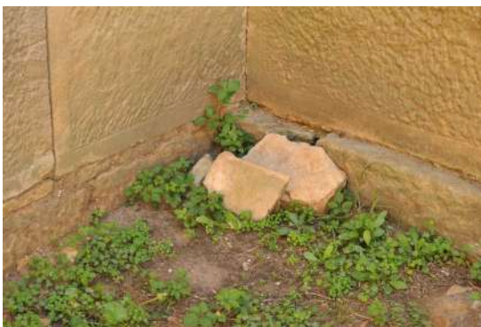
Figure 73: View of recent delaminated stone blocks on the western elevation.
