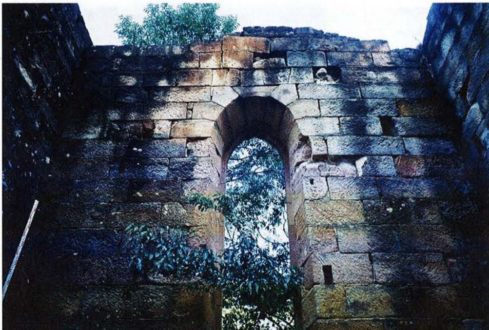
Figure 9: The walls of the south front porch are substantially thicker than the nave walls suggesting that a tower or spire had been originally planned atop the porch. The photograph shows evidence of notched stonework to support a floor and a stair or ladder (photograph: John McInnes, Nov. 2002)
