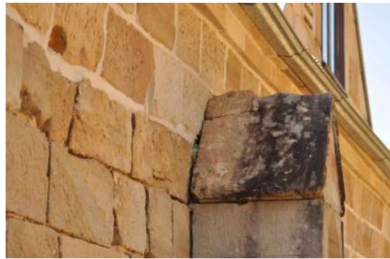
Figure 78: View of the mortar joint failure on the western elevation.
