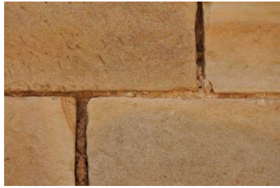
Figure 82: Typical View of the deteriorating shell lime mortar joints.
