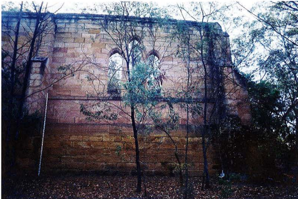
Figure 8: Section of east elevation showing intact triple lancet window, stringcourse and engaged buttresses. (Photograph: John McInnes, November 2002)
