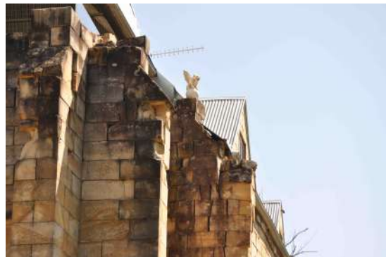
Figure 70: View of the buttresses on the eastern elevation showing missing fabric and displacement of stone blocks.
