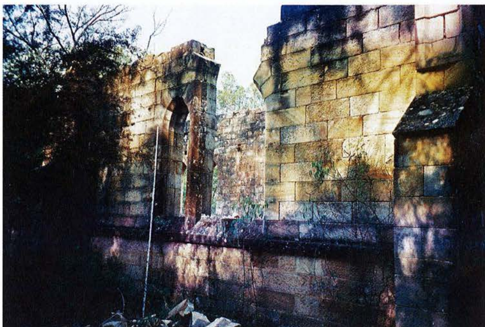
Figure 7: Photograph of west wall showing collapsed stone around window, stringcourse, buttress treatment, half course and fine ashlar masonry. (Photograph: John McInnes, November 2002)
