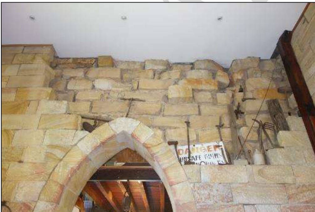
P08 – HISTORIC COLLAPSE OF INTERNAL DIVIDING WALL (NOT REPAIRED)
