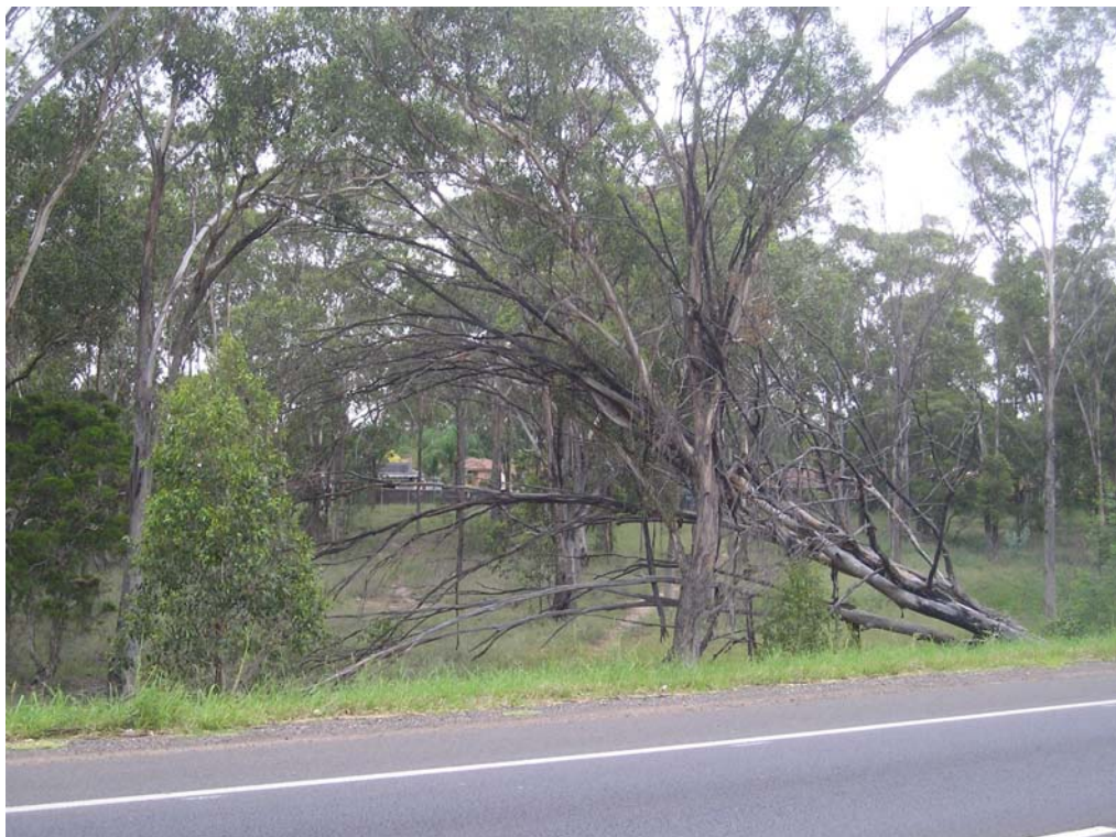
George Street Embankment (north end) with fallen trees due to undermining by water flow and inappropriate drainage design, Reserve #116..
