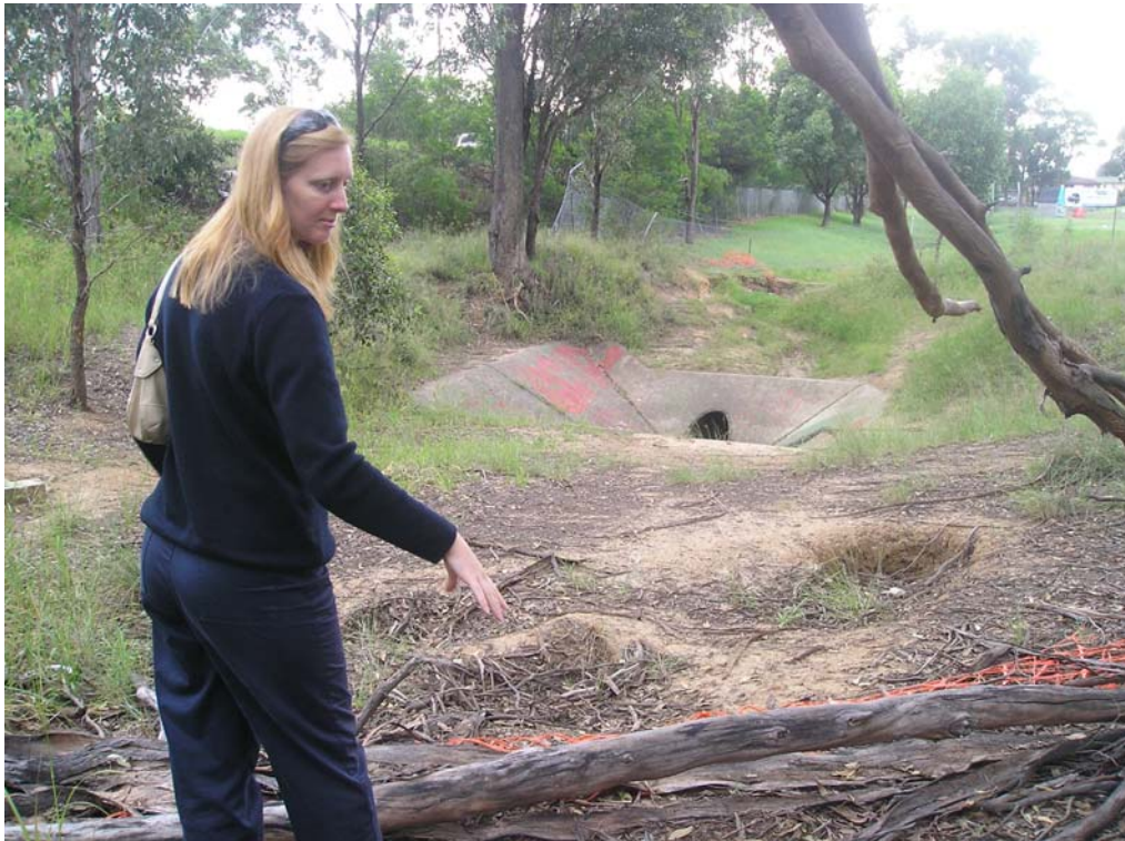
Pipe erosion, subsidence and other major drainage problems in Reserve #116 – north-western corner near Rugby Leagues Club Ovals. Note collapsing fence and fallen trees on embankment.
