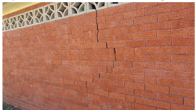
Existing amenities building that needs to be demolished
