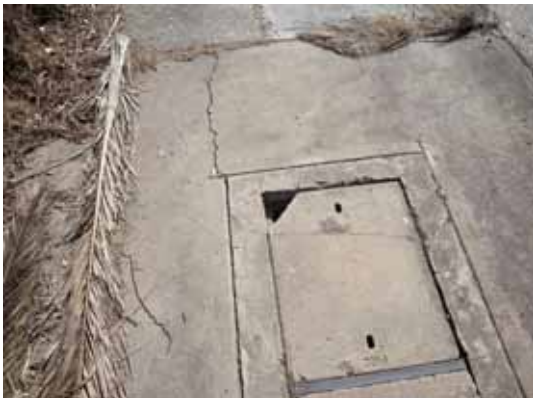
Figure 8.4: Damaged service pit in footpath
