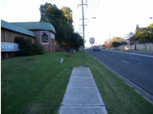
Figure 8.12: Lack of connectivity between footpaths
