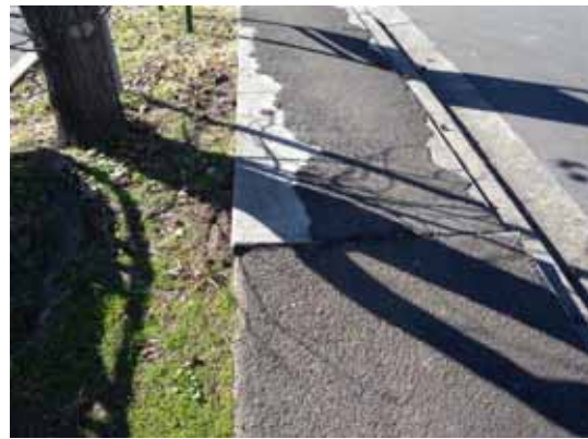
Figure 8.11: Narrow kerb ramps – pedestrians directed towards traffic
