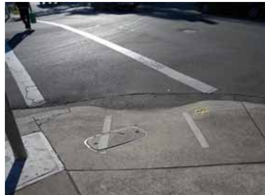
Figure 8.5: Kerb ramps at intersection – incorrect alignment
