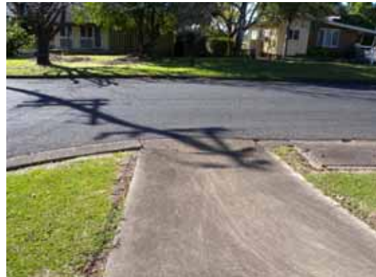
Figure 8.7: Kerb ramps on only one side of a street
