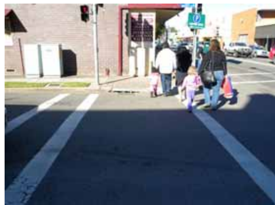
Figure 8.11: Narrow kerb ramps – pedestrians directed towards traffic
