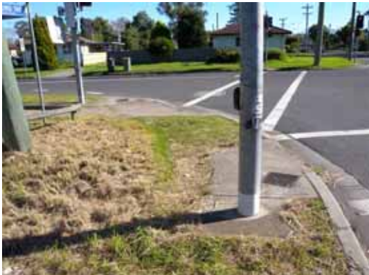
Figure 8.6: Disjointed kerb ramps at an intersection
