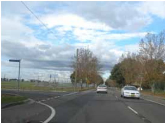
Figure 5.8: Unsatisfactory Intersection Linemarking
