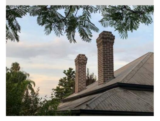
Damaged chimneys needed repointing.
