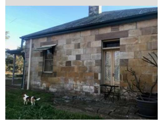
To prevent further fretting of this wall and the sandstone chimney, replacement of the existing cement mortar with lime based mortar was needed.
