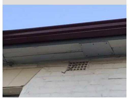
Minor maintenance was needed to replace badly deteriorated timber eaves.
