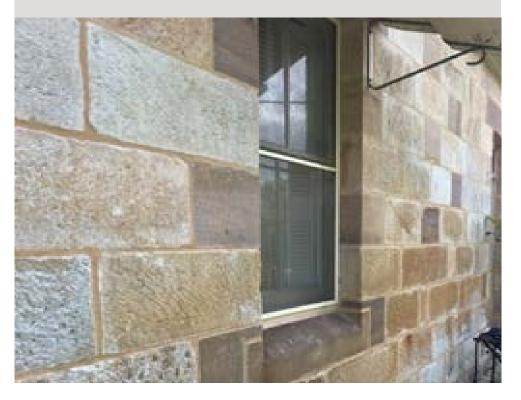
Repointed wall with lime based mortar with the correct mixture prevents further fretting. The completed works provide improved protection to the wall.
