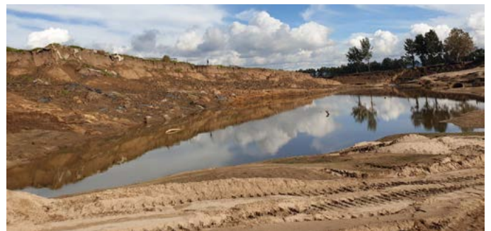
Cornwallis flood mitigation repair earthworks
