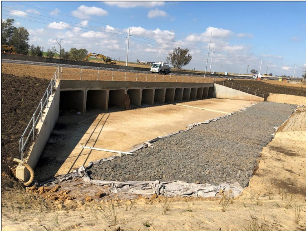
Figure 30 Multi-cell box culvert under construction
