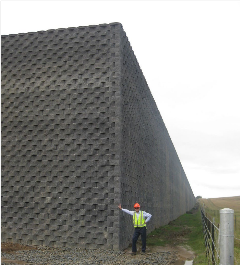
Figure 24 Industrial Retaining Wall, Horsley Park, Fairfield City
