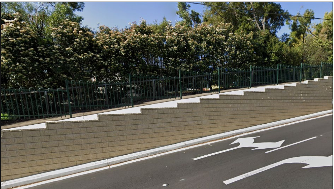
Figure 23 Roadside retaining wall Glenhaven Road, The Hills Shire
