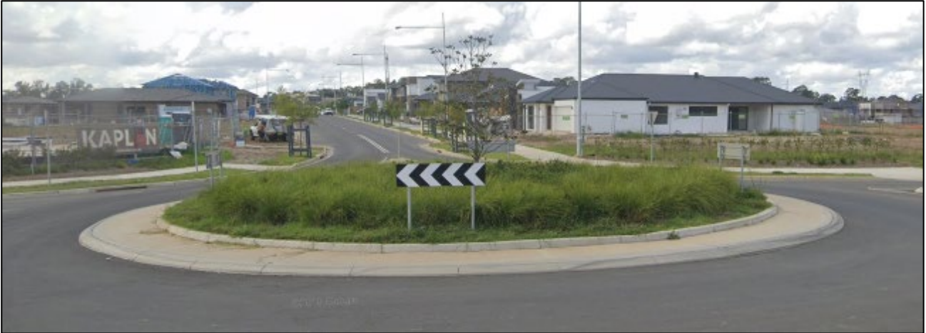
Figure 13 Recently installed landscaped roundabout in Camden
