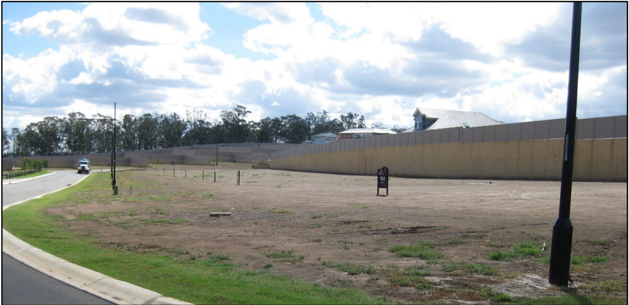
Figure 1 Retaining walls for new lots
