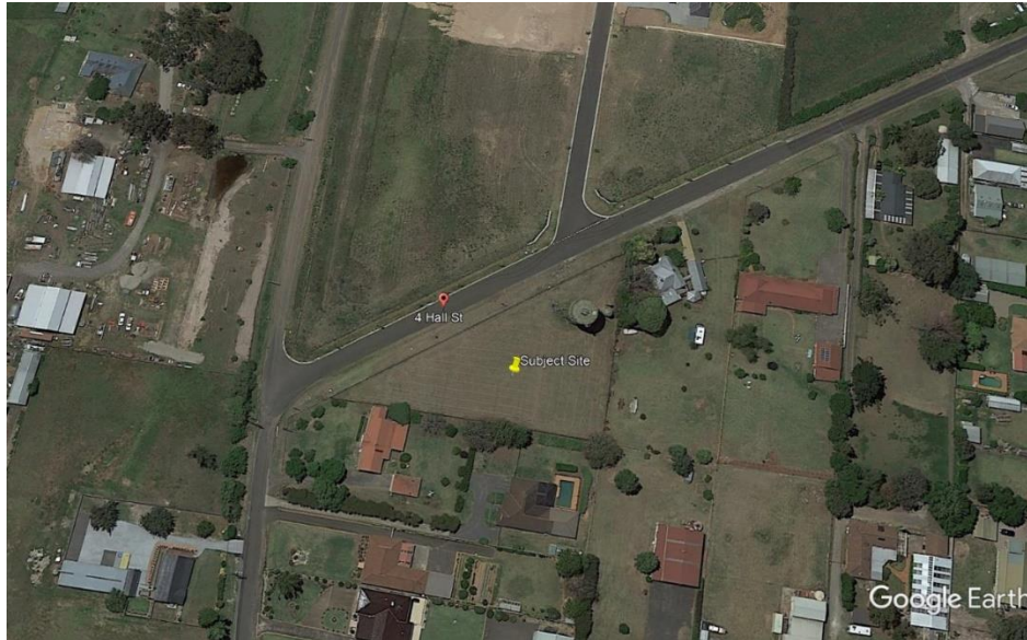
View of subject site
