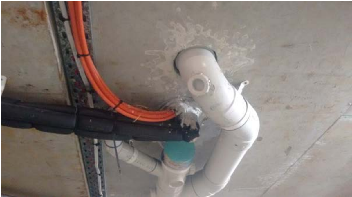
Figure 9: Pipe penetrations that are not appropriately protected with fire collars. This work appears to be recently carried out. There is no evidence of an approval having been issued.
