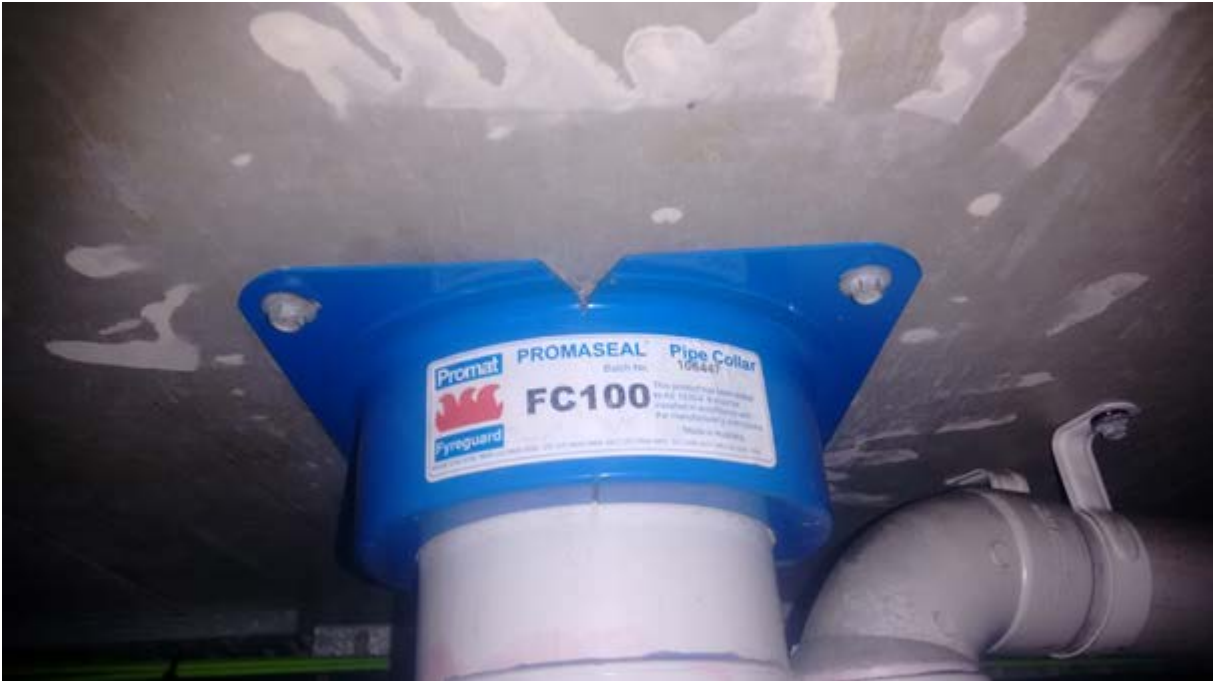
Figure 7: A retro-fitted fire collar to a pipe penetration through the concrete slab.
