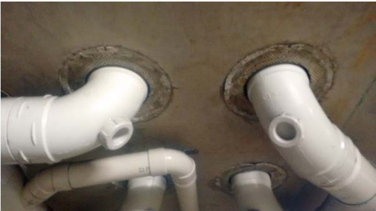
Figure 8: Fire collars cast into the slab during construction.
