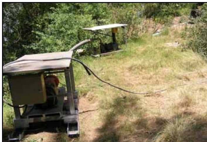
PHOTO 13: The southern portion of the reserve (river bank) contains a number of irrigation pump-sites and piping, overground electrical cabling and unsecured meter boxes on elevated towers. This infrastructure, currently under licence or permissive occupancy on the Crown reserve, raises issues over public safety and risk management. These issues need to be addressed in accordance with this plan of management.
