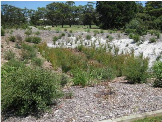
**Figure 3-5 Example of a Bioretention System**
