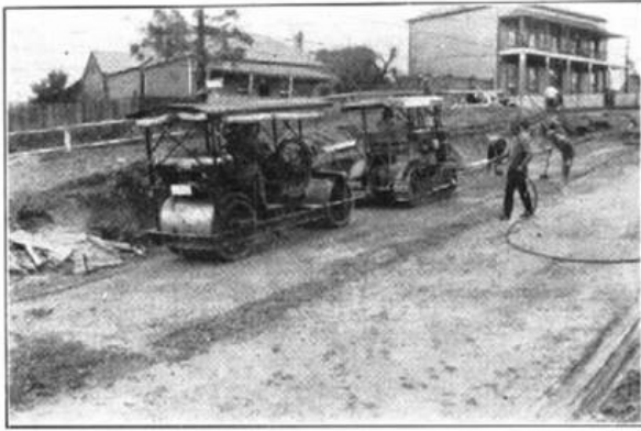
Fig. 1. Connecting road Windsor. Tractor towing roller.
