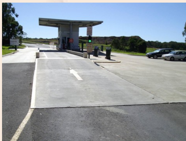
Weighbridges at the Hawkesbury Waste Management Facility
