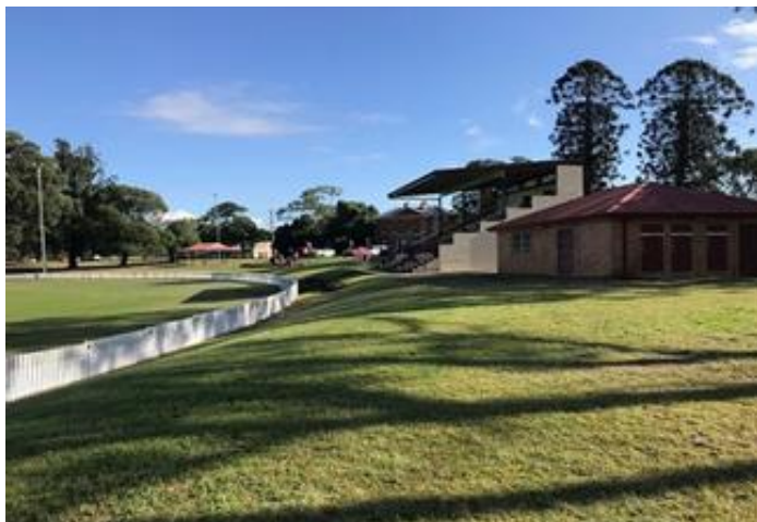
Photo 5: View looking north over McQuade Oval, grandstand & amenities block/ kiosk. Heritage Bunya Pines [b/g] (29/05/2020).
