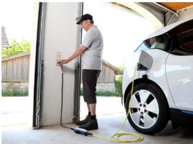
Figure 15: Making homes EV ready
