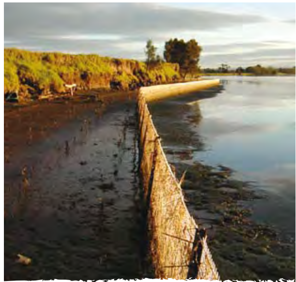
Mangrove seedlings planted in front of an eroding bank along the Shoalhaven River, with the use of temporary mesh fencing as a wave barrier. Photo: Allan Lugg, Department of Primary Industries.
